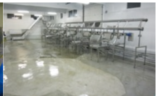
Floe-line with 6 work stations
