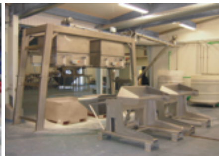
Double Salt Spreading Line
