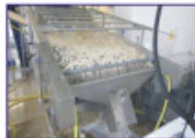
Scallop processing plant
